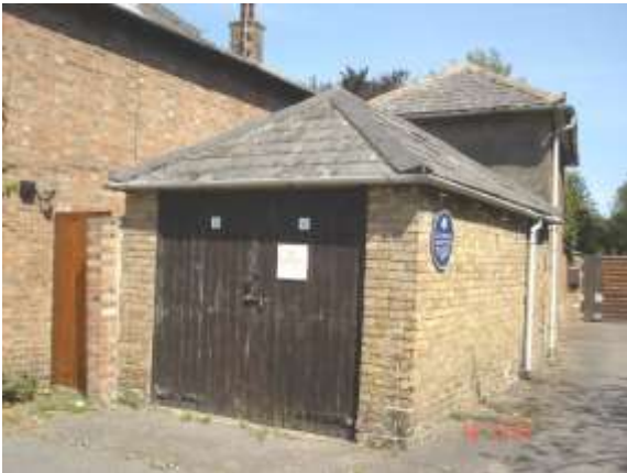
Fire Pump Accommodation
