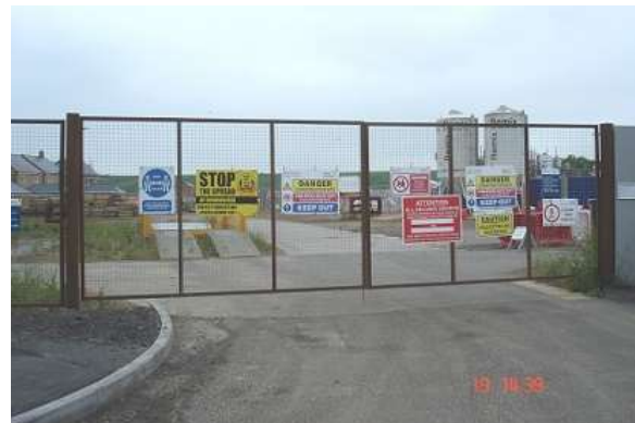
295 Bovis Homes under construction in 2022
