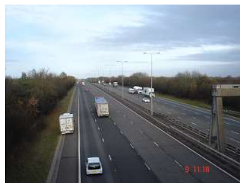
The A1M from St Andrew's Flyover
