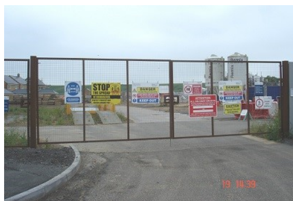
295 Bovis Homes under construction in 2022
