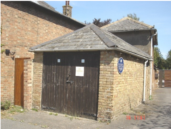
Fire Pump Accommodation
